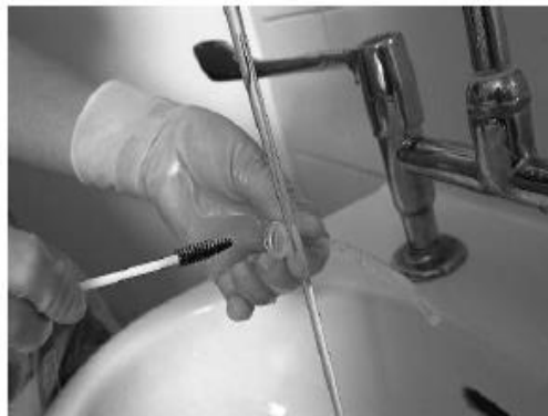
Fig. 4: Removal of the inner tube.
